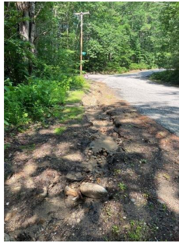
View of the road shoulder erosion along Long Pond Road near Pine Street.
